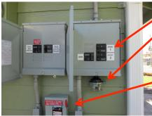
All circuits are clearly labeled. Each PV system includes a lightning arrestor, which protects the equipment in the event of a voltage spike. Non-stainless steel unpainted parts are coated with UV resistant clear enamel.
