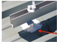
On nearly flat roofs, when the penetrations are sealed to specification, another layer of sealant is applied, such as the elastomeric coating shown in the adjacent photos.
