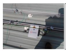
Exterior ground connections are made using insulated wire to prevent contact between 2 dissimilar metals. Where the wire is stripped it is coated with Scotchkote so that moisture cannot bridge the materials.
