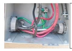
All conduits running between junction boxes and switch gear are plugged with duct seal putty. This reduces the possibility of humidity or critters migrating from device to device.
